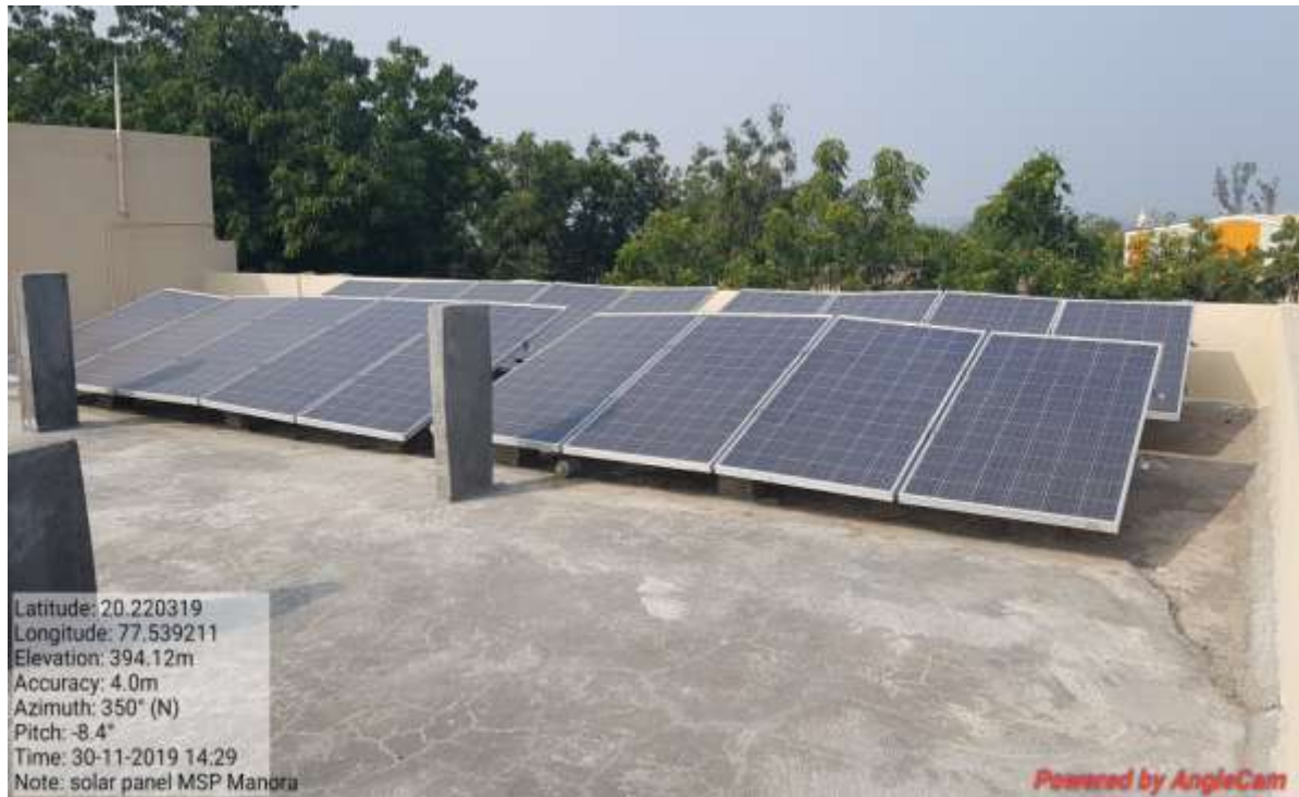
Photo: Solar panel(5.5 kW) on the roof of hostel building
