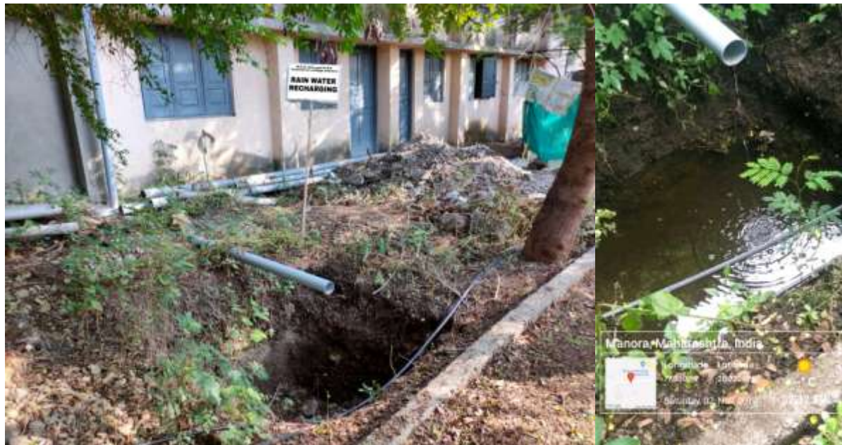
Photo: Showing down water pipe system for Recharging of rain water behind Library
